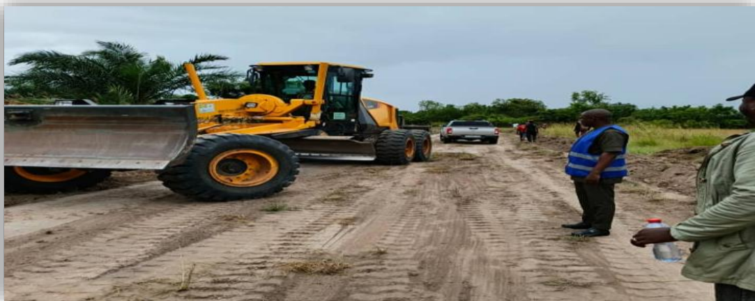
Reshaping of roads in the District
